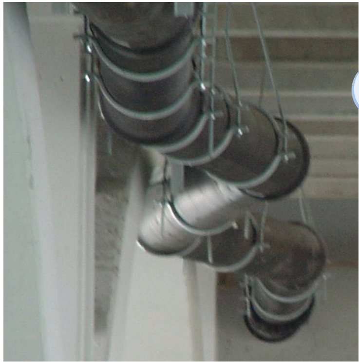
Pipeline “Snaking” Due to Inadequate Lateral Support
